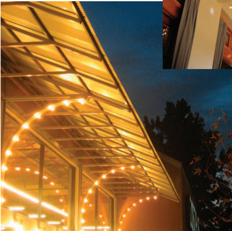
This metal-bracketed overhang is lit with multiple lights, producing multiple reflections on surfaces.
