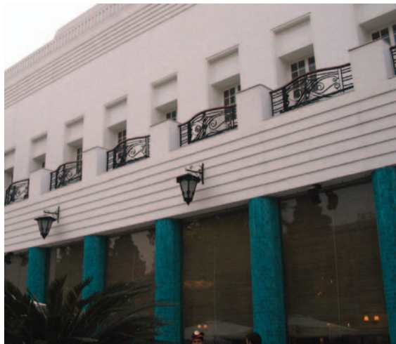
Smaller upper level openings follow the rhythm of larger openings below.
