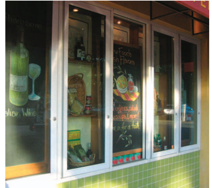
Shallow display shelves (within the exterior wall thickness) with exterior opening windows for access allow full use of the interior space.
