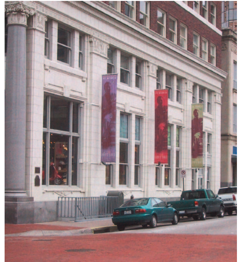
Use of banners mounted on pilasters creates an additional architectural element on the building facade.
