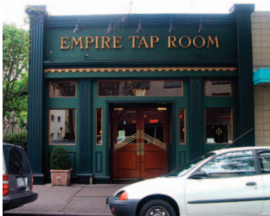
Covering the entire facade with storefront treatment is most effective for small one-story buildings.
