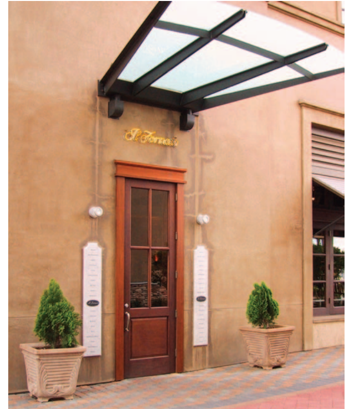
Canopies are made with attractive lightweight roofs.
