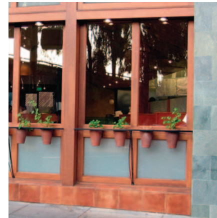
Translucent glass treatment with landscaping compensates for full-length glazing.
