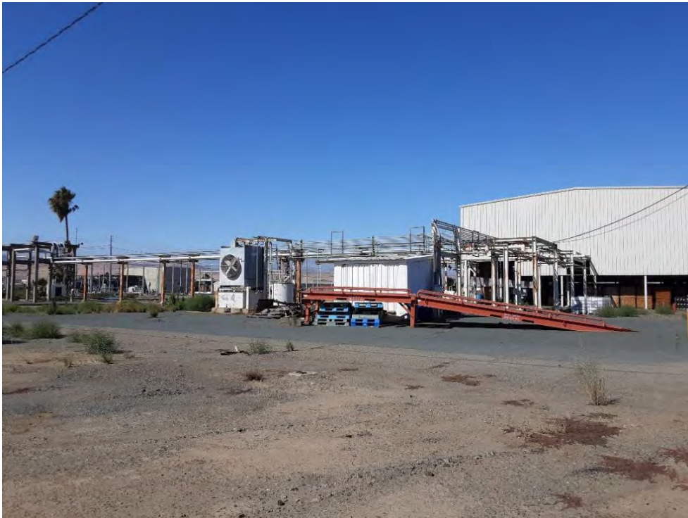
Photo 4: Site overview – looking southwest (Photo Date 8/25/2023)
