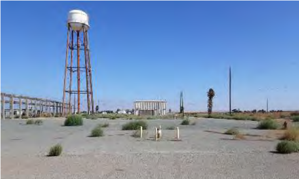
Photo 13: Site overview of northeast section of Project existing conditions.
