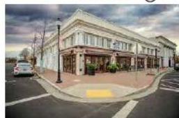
444 RAILROAD AVE. ⑤
