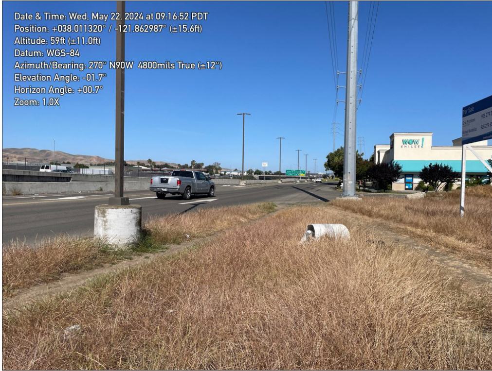
Photo 5. Trash and debris were observed onsite located within the southwest portion of the site, with North Park Boulevard seen on the lefthand side of the photo. Facing in the west direction.
