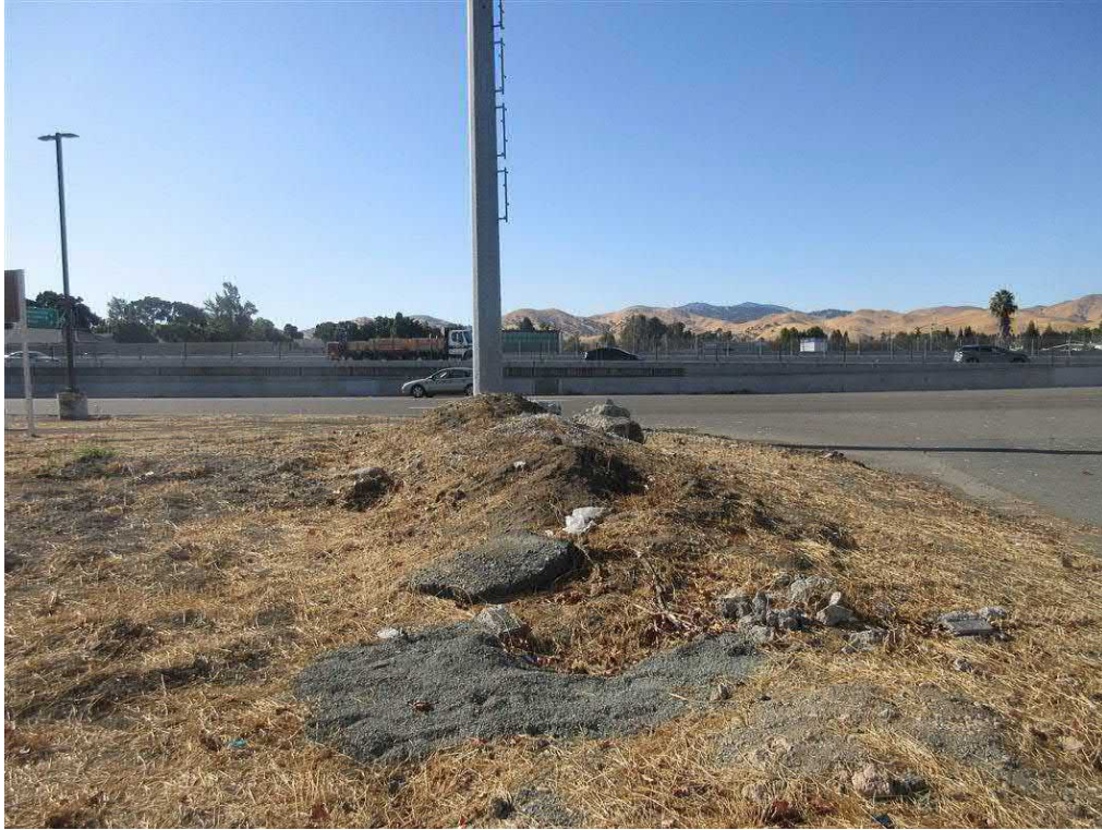
Photo 11: Southern-facing view of the apparent end-dump soil and debris piles located in the southwestern portion of the subject site.
